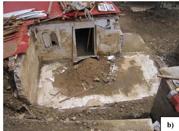
Figure 4: Perspective views of the a) mud flow that caused extensive damages to b) Ampliani's village buildings.
